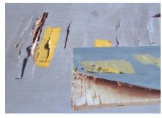
Extensive substrate failures and "alligator skin cracks" were evident throughout this job site before the poly-deck was replaced.
