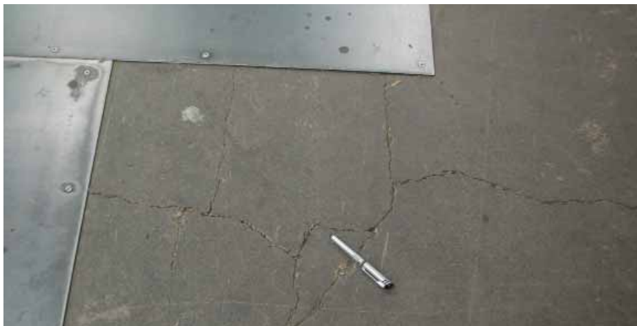
Prior to ResinDek repair, steel plate had to be attached on top of the concrete mezzanine floor so pallet truck wheels could continue to roll
