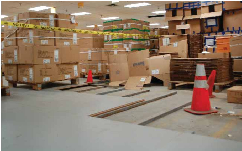
Installation of ResinDek and steel sleepers over damaged concrete
