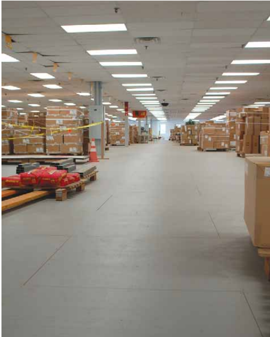
New ResinDek® panels installed
